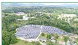
Kearsarge Pittsfield (Pittsfield, MA) – 1.9 MW
