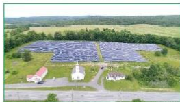
Kearsarge Windsor (Windsor, MA) – 1.4 MW
