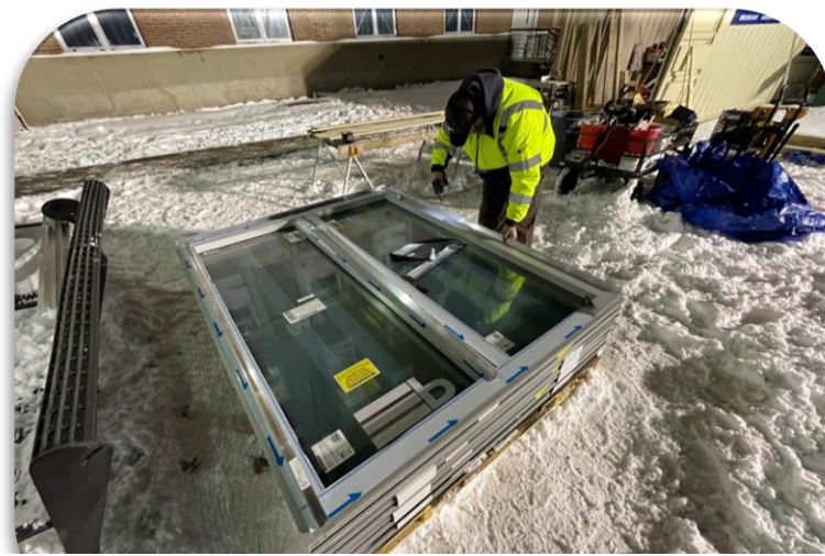
Windows being installed at the High School of Sci-Tech
