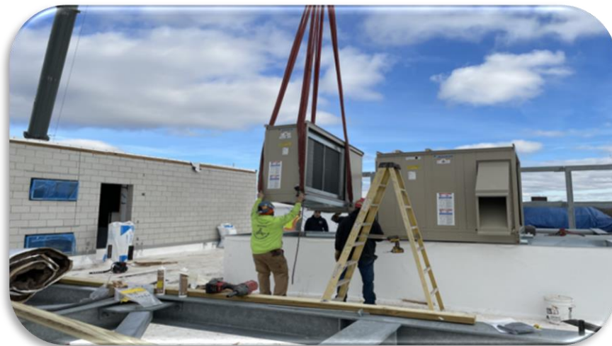
Air Handling Unit (AHU) being installed at DeBerry-Swan School
