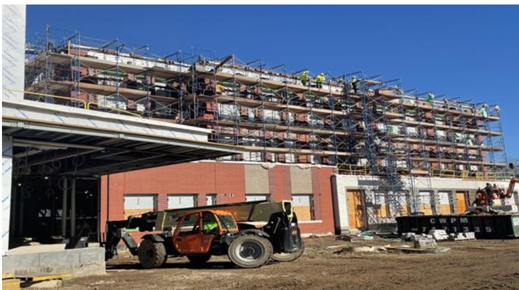
(DeBerry-Swan School Construction: October 2022)
