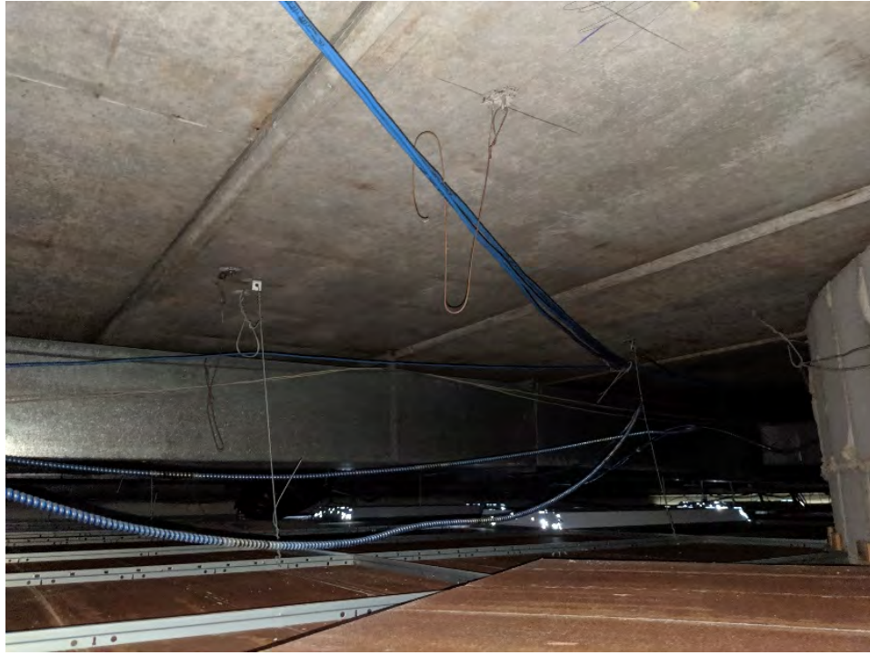
PHOTO 21: TYPICAL CONDITION OF UNDERSIDE OF PRESTRESSED CONCRETE BOX BEAMS
