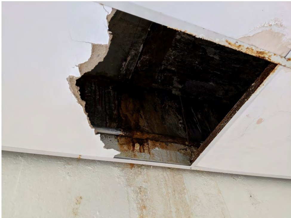
PHOTO 28: RUSTED UTILITY CONDUIT BETWEEN BEAMS 2 AND 3 AT SOUTH ABUTMENT
