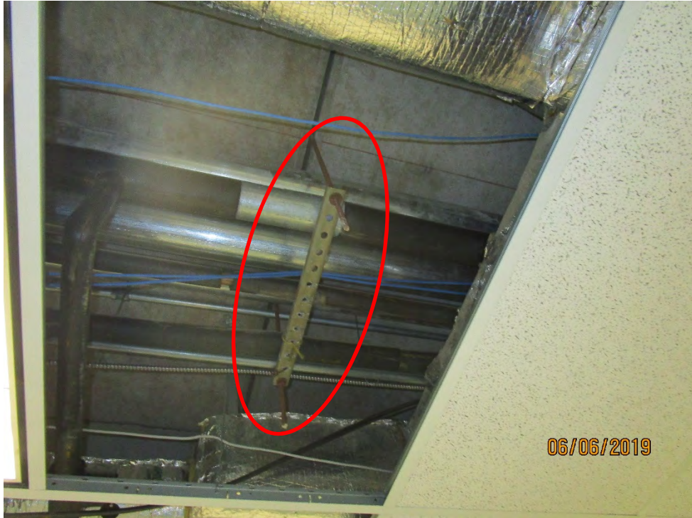
PHOTO 11: UTILITY ANCHOR ROD INSTALLED IN JOINT BETWEEN BEAMS 11 AND 12
