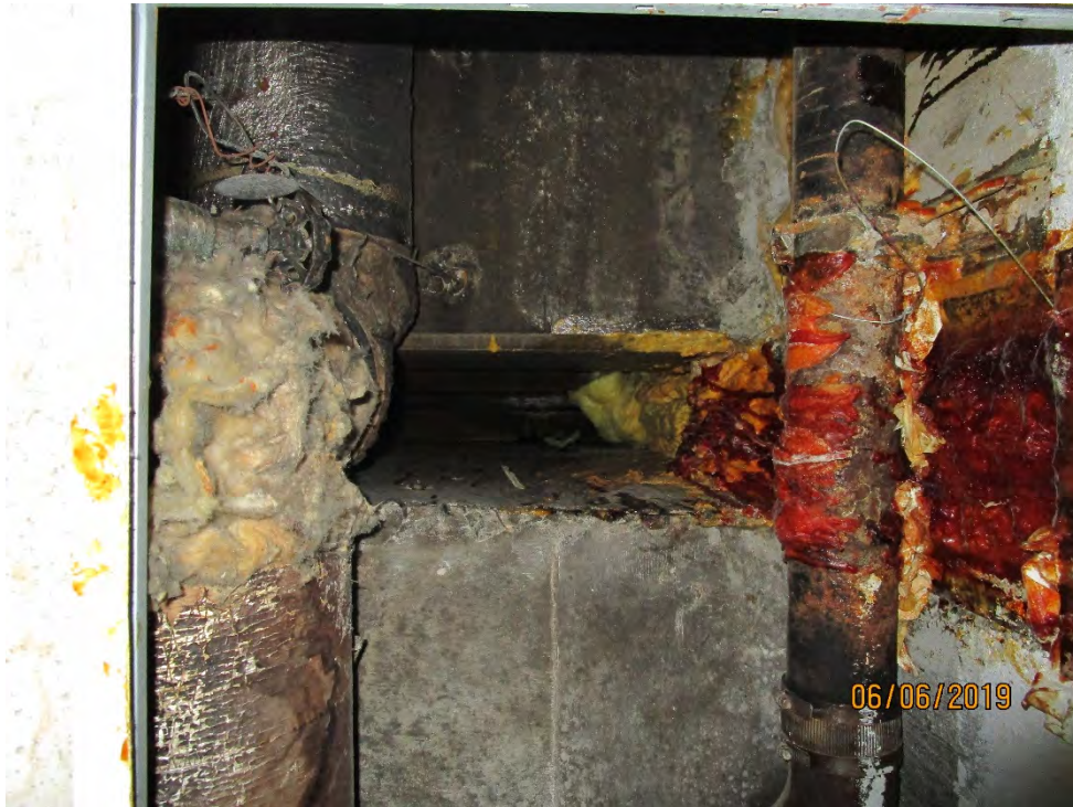
PHOTO 17: WATER INFILTRATION BETWEEN EDGE BEAM 1 AND PRESTRESSED BEAM 1
