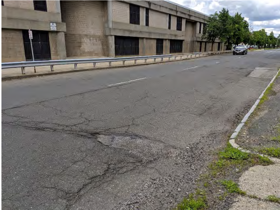
PHOTO 35: BIRNIE AVENUE OVER BRIDGE LOOKING NORTH
