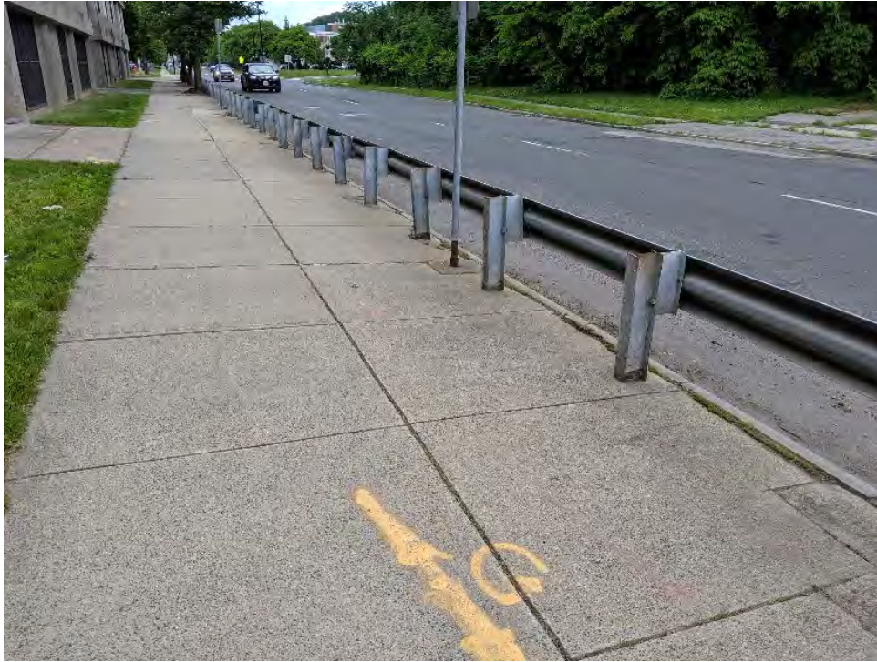
PHOTO 37: WEST SIDEWALK ON BIRNIE AVENUE AT BRIDGE FACING NORTH
