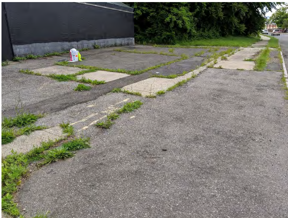
PHOTO 32: PAVED AREA OVER BRIDGE EAST OF BIRNIE AVENUE
