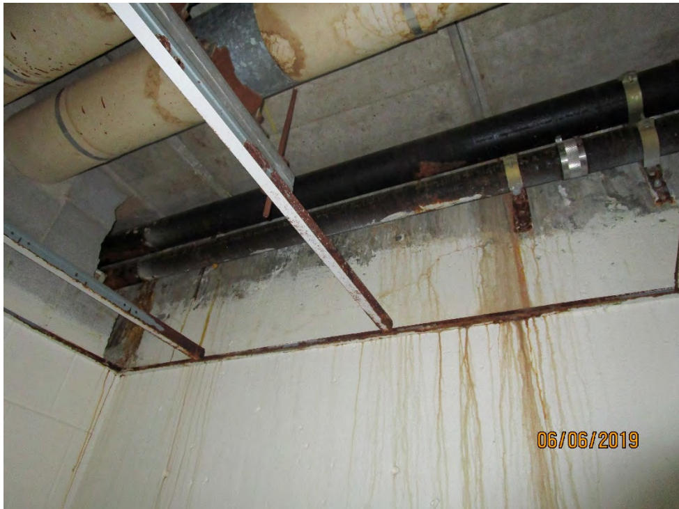
PHOTO 6: UNDERSIDE OF BEAMS 20-22 AT NORTH ABUTMENT
