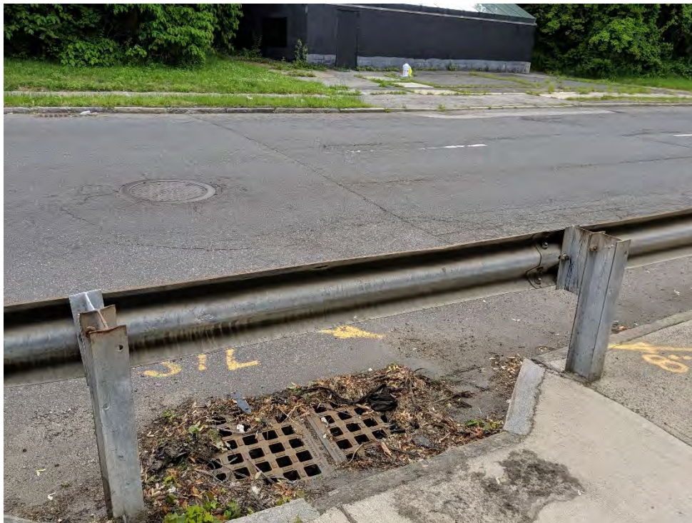
PHOTO 38: STORM DRAIN ON BIRNIE AVENUE AT NORTHWEST CORNER OF BRIDGE
