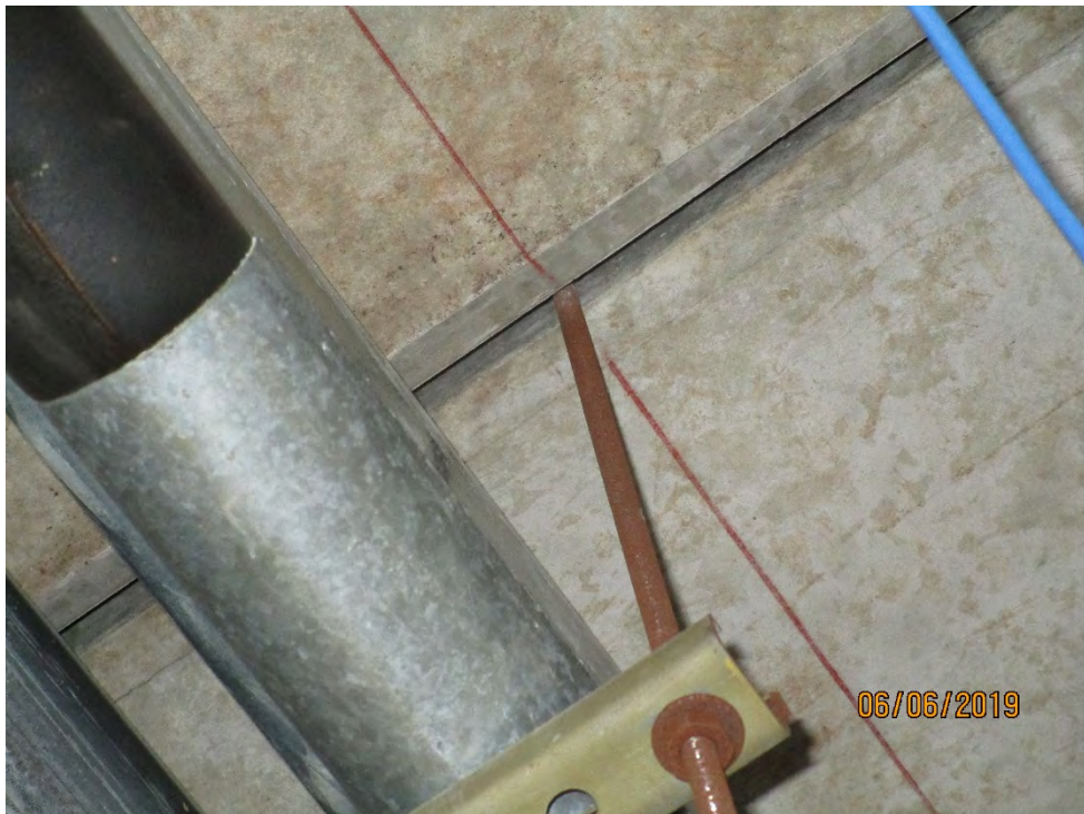
PHOTO 12: UTILITY ANCHOR ROD INSTALLED IN JOINT BETWEEN BEAMS 11 AND 12 (CLOSE-UP)
