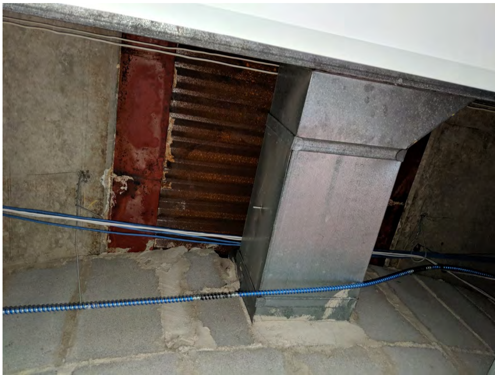
PHOTO 22: UTILITY BAY BETWEEN BEAMS 17 AND 18
