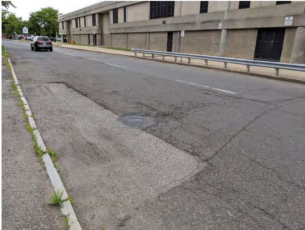
PHOTO 31: BIRNIE AVENUE AT BRIDGE LOOKING SOUTH
