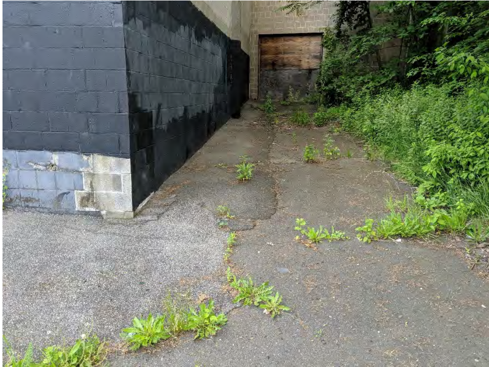
PHOTO 33: VIEW OF ATRIUM FACING EAST
