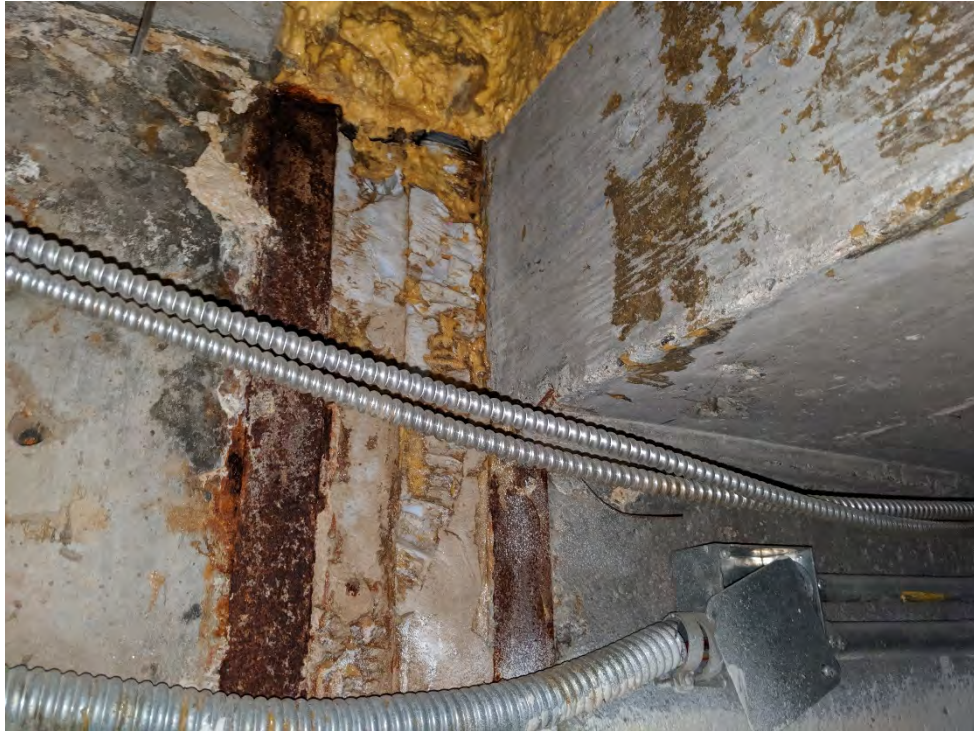
PHOTO 25: SOUTHWEST CORNER OF SOUTH ABUTMENT EXPANSION JOINT
