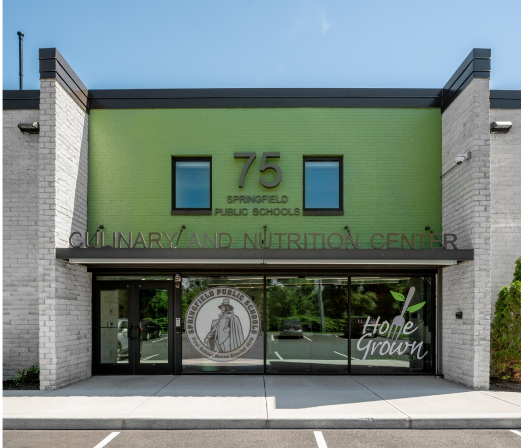
The new Springfield Culinary and Nutrition Center, located on Cadwell Drive.
