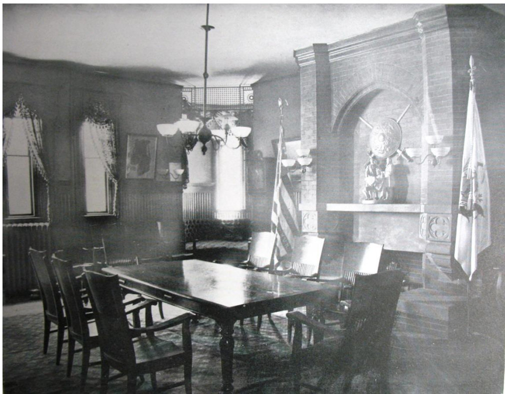
Figure 8: Second Regiment headquarters room, with distinctive fireplace, c. 1899. 11
