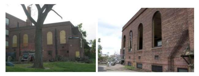
The brick parapets were blown off entirely at the south end of the main building and the lower portions of gym building had large sections of brick removed. These lower structures looked to be disconnected (not toothed-in) to the main gym structure and have been displaced.
