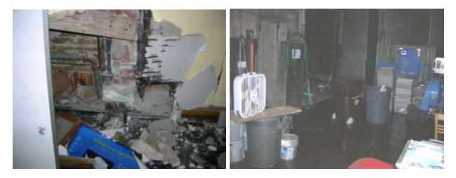
Since power was lost to the building during the storm, certain systems could not be observed to confirm their integrity. The loss of power did cause a failure of the basement sump pump which led to flooding of the basement; about 1"-2" of ground water was standing in the basement at the time of the professional team's visit.
