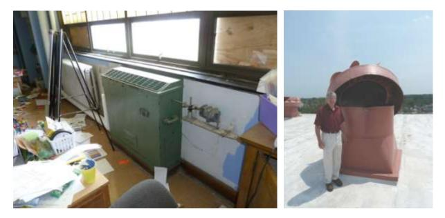
The rooftop ventilators, although re-installed, are damaged and probably not salvageable. Also rooftop condensing units appear to have been displaced and are probably damaged.
