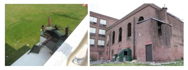
The main roof also suffered damage in several isolated areas caused by wind-blown debris which tore the membrane or was imbedded in the layers of insulation.
