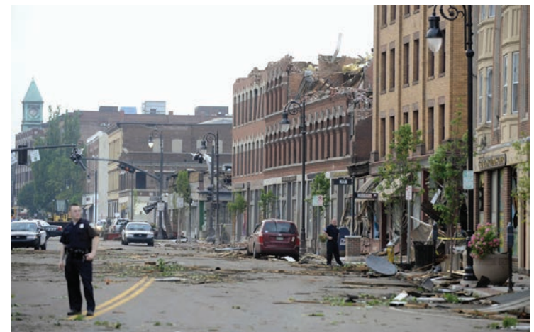
Tornado damage at Main and Hubbard Streets
