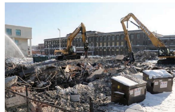
Union Station Under Construction
