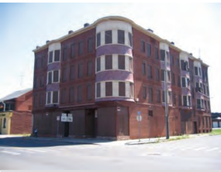
286 Main St/11 Spring St, Holyoke. This vacant building includes 15 units and has been on the market for over a decade at $600,000. Source: City of Holyoke
