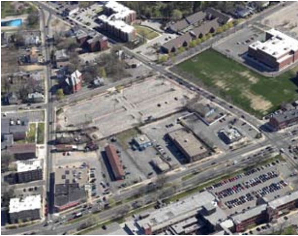
The Walnut-to-Oak Block with State Street in the foreground.
