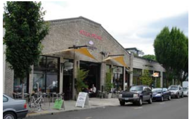
Results of a façade-improvement program in Portland, Oregon.
