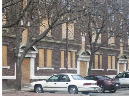
Hollywood vacant apartments
